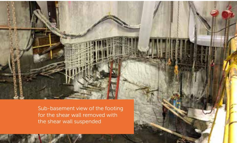
Sub-basement view of the footing for the shear wall removed with the shear wall suspended
