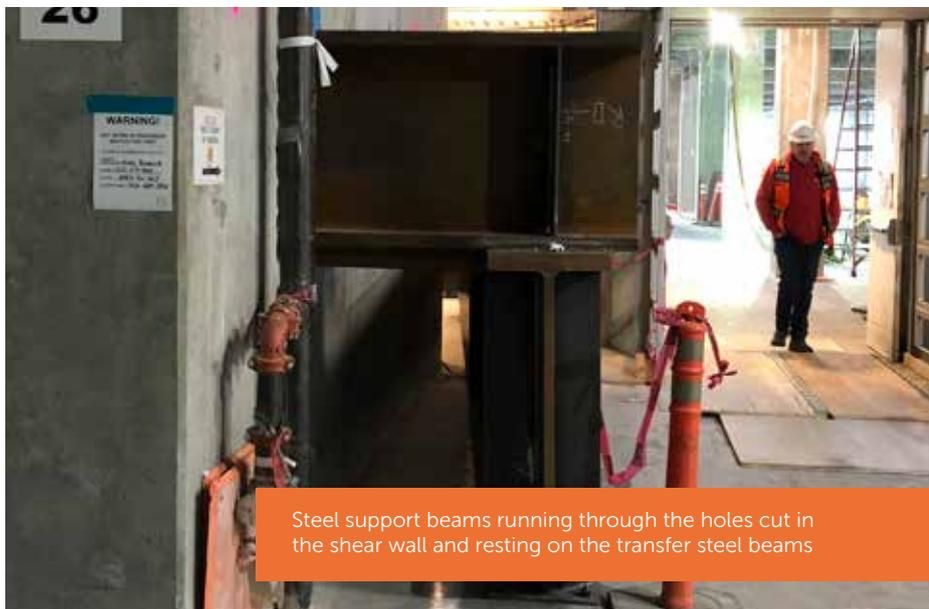
Steel support beams running through the holes cut in the shear wall and resting on the transfer steel beams
