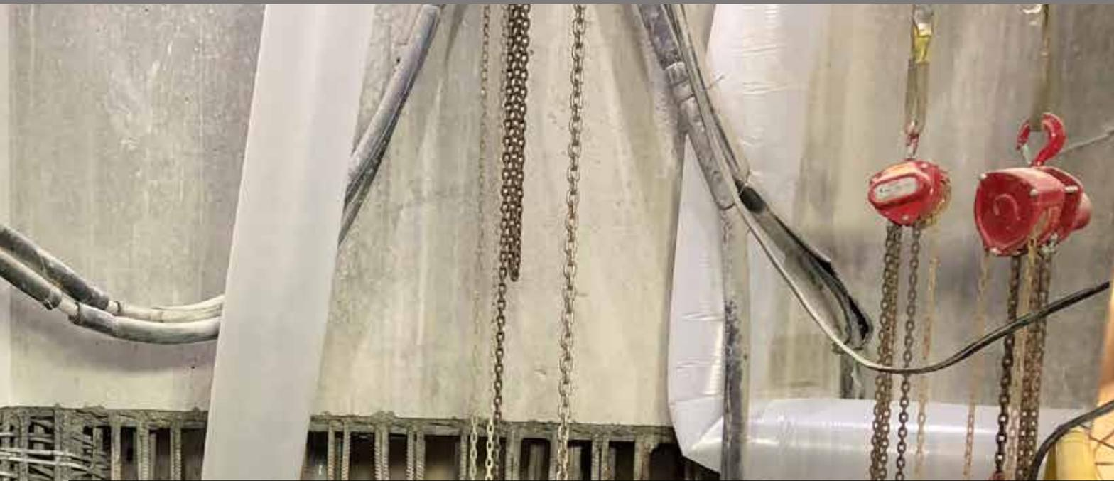
**T**his project began when GLY Construction was approached by their client with a challenging request that seemed nearly impossible in the beginning, to create a shoring system to fully support the disconnection of a shear wall from the foundation. The request was to take an existing C-shaped shear wall/elevator shaft that was approximately 80 feet tall and 2 feet wide and rotate it 90 degrees. In order
