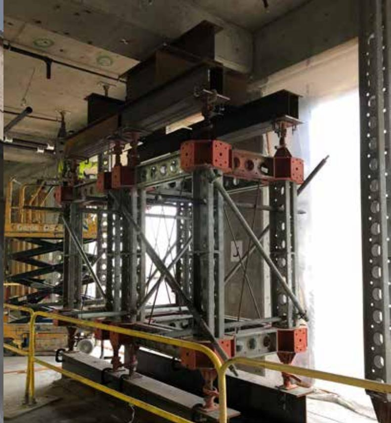
must remove column, therefore must support beams attached to column), it is vital to take a holistic view of any demolition concept. What may appear to be a straightforward shoring project could become increasingly complex when having to consider the loads of upper floors. In the case of multi-level buildings, any column removed on a lower floor will have a direct impact on the floors above, magnifying and potentially multiplying the loads that need to be supported.
