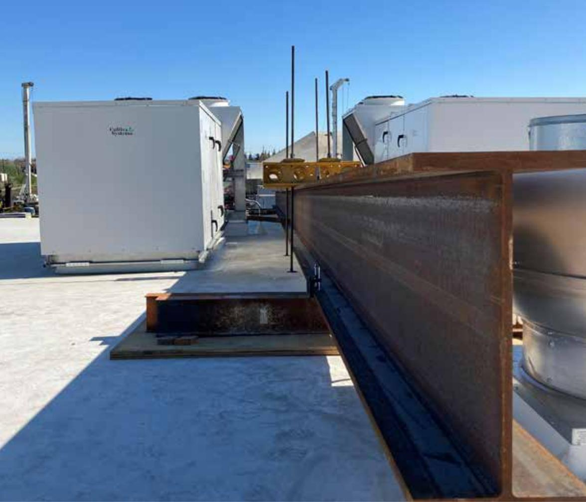
shoring beam was craned onto the roof and into position directly above the damaged roof girder.
